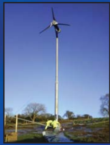
Photo shows the turbine being installed.
